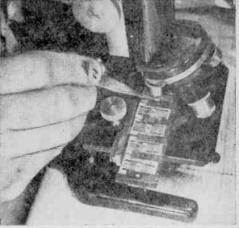
You can expect the assembly of mini amps to be partially executed under a microscope. After this amplifier is done it will be sealed in helium to prevent deterioration.
